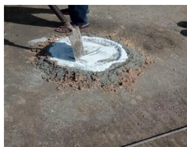
(b) Cement and recycled glass powder added to fine aggregates
