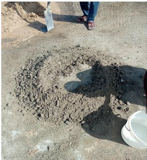
(f) Water added to the mixture of fine aggregate, cement, recycled glass powder, coarse aggregate, and palm kernel shells
