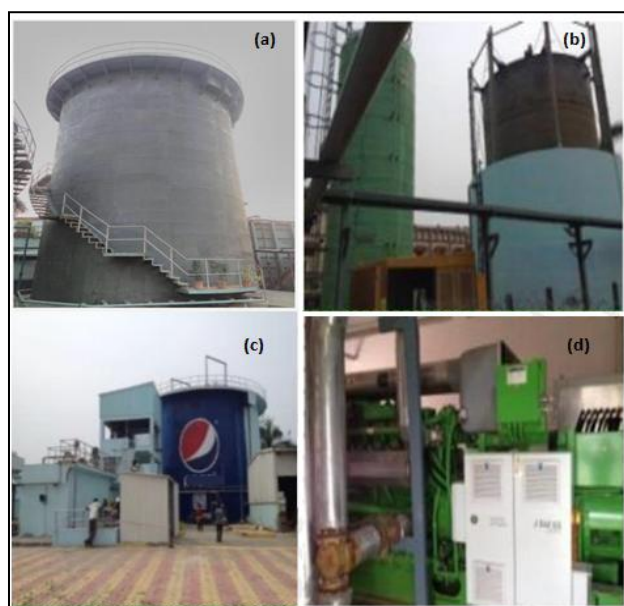
Fig. 5. Industrial set-up for bio-methanation (a) Pre-treatment with Up-flow Anaerobic Sludge Blanketing reactor (UASBR), (b) Gas holding tank, (c) Collector, (d) Methane to Electricity generator
