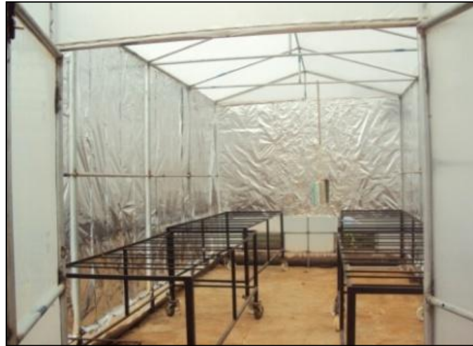
Fig. 2. Modified Solar greenhouse dryer using aluminium foil on eastern, western and southern walls
