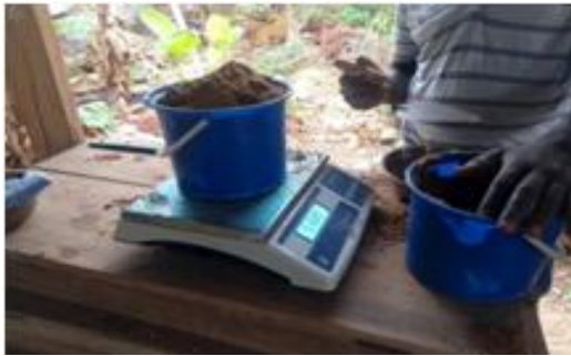
Fig. 4. Batching process of the constituent materials
