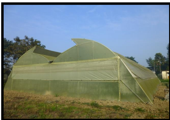
Plate 1. Showing site view
