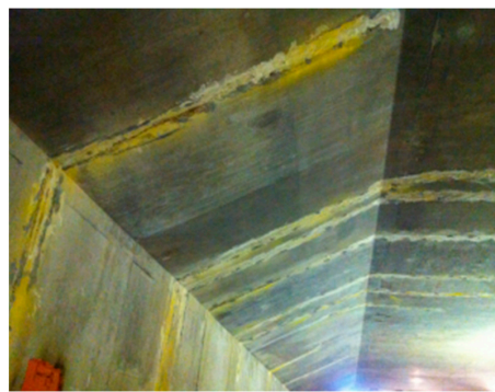
Figure 14. Tunnel patch processing site diagram.
