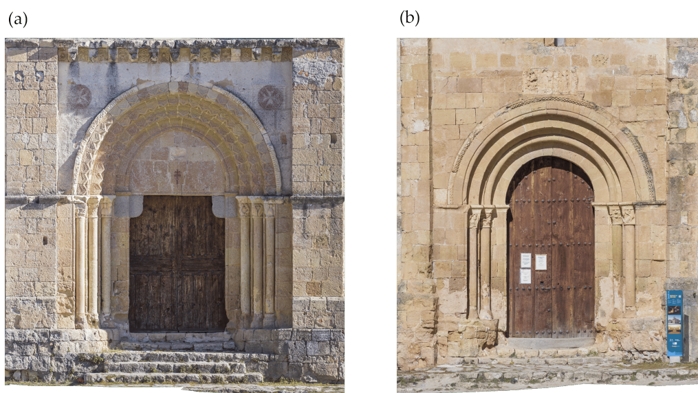
Figure 2. Church façades: (a) West doorway; (b) South doorway. Orthoimages: Luis-Javier Sánchez-Aparicio.
